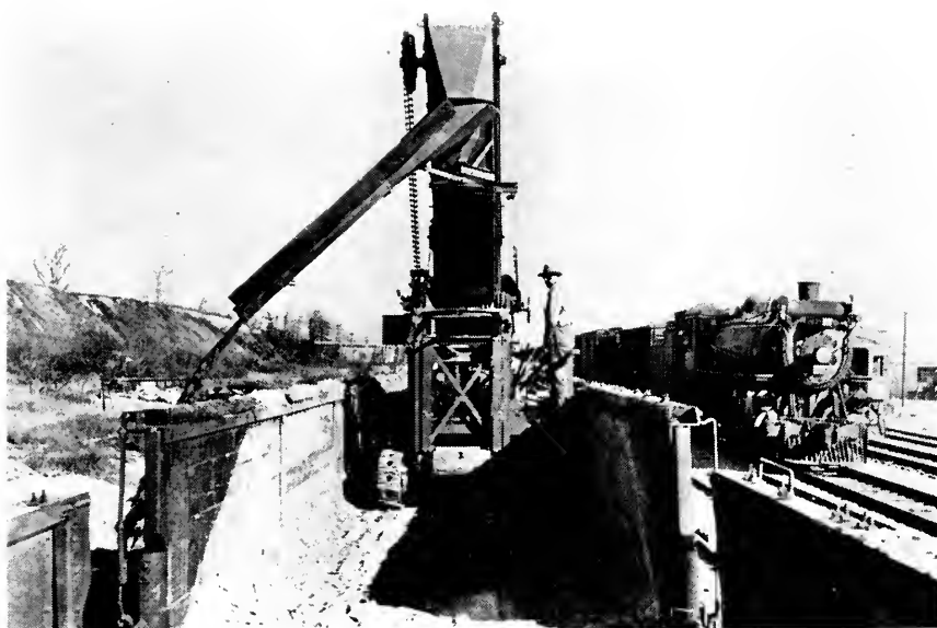
Conveyor-type bucket loader being used to unload ballast.
